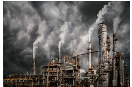
Hazardous material response
